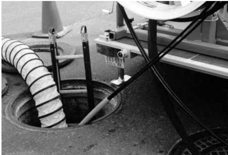
Figure 7-7 Two fiber optic cables being pulled through innerduct that has previously been pulled into conduit. Courtesy Condux
